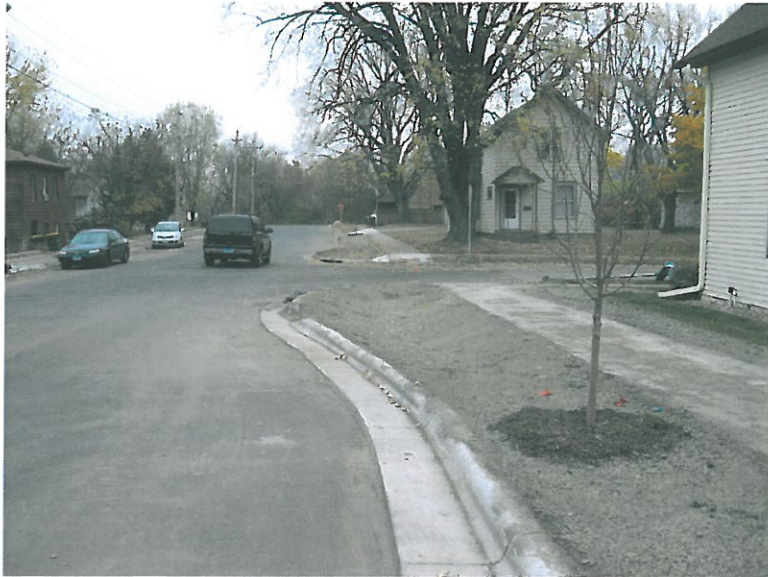
Photograph above: one depressed “bump-out” used to collect street runoff.
