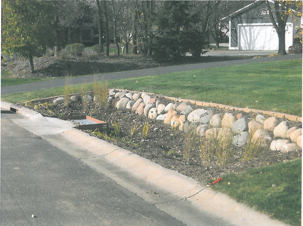
Photograph of raingarden on Nena Drive, which overflows to Amundson Drive.
