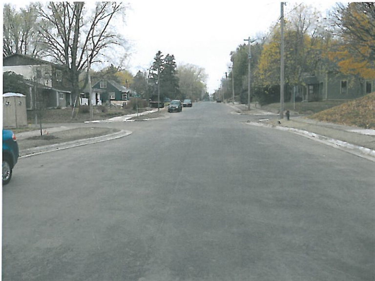
Photograph above: street view of several “bump-outs” on Wilkins Street.
