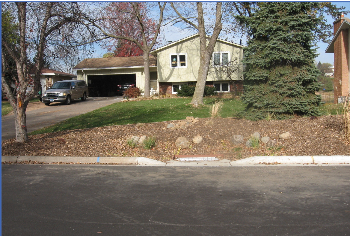
Completed bioretention cell, October 2011. Inlet pretreatment box chamber prevents debris and sediment entry into the bioretention cell. Lake McKusick is visible in the background.
