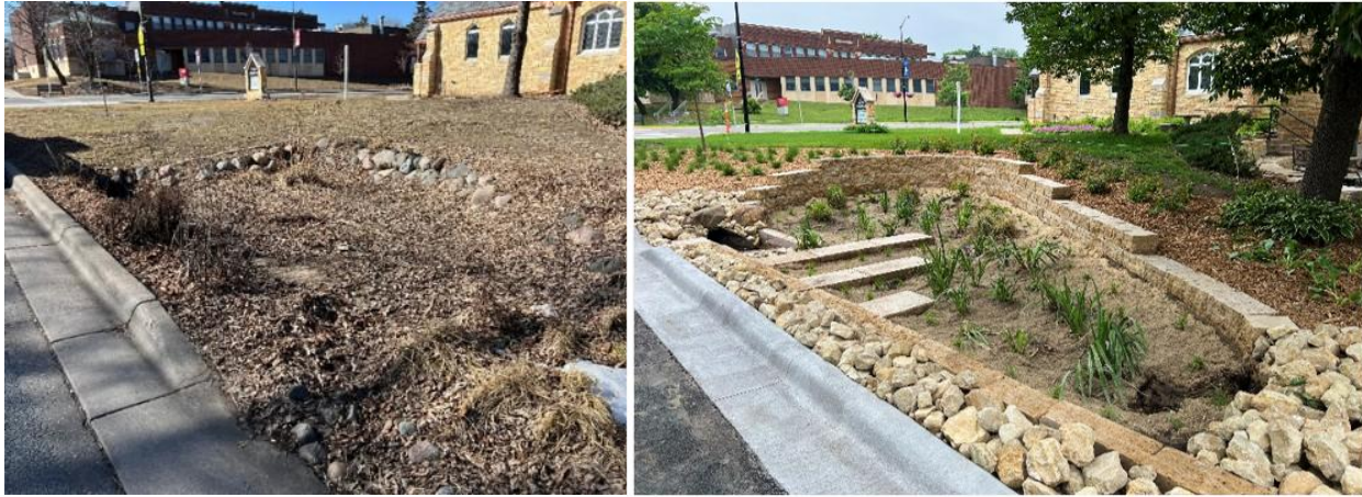
[Above] Before (left) and after construction (right).
