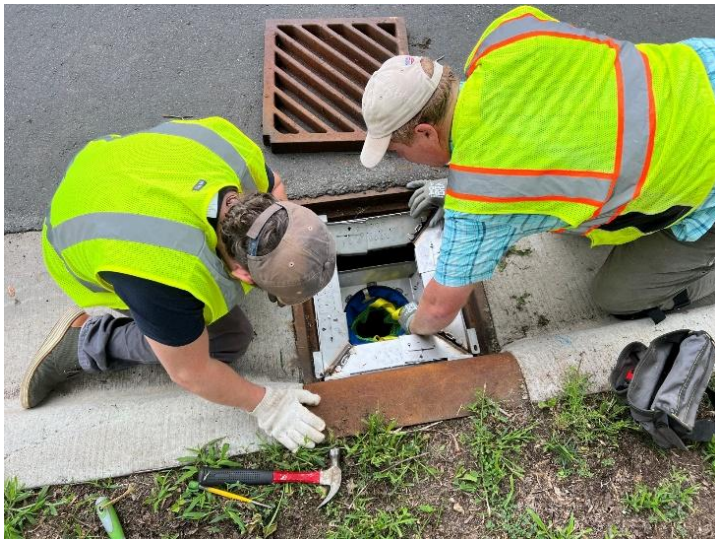
[Above] CSAH 5/Owens St N Gutter Bin installation, Stillwater.
