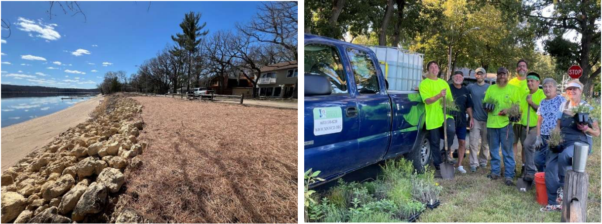
[Above] Section 5 stabilization, upland buffer restoration.
