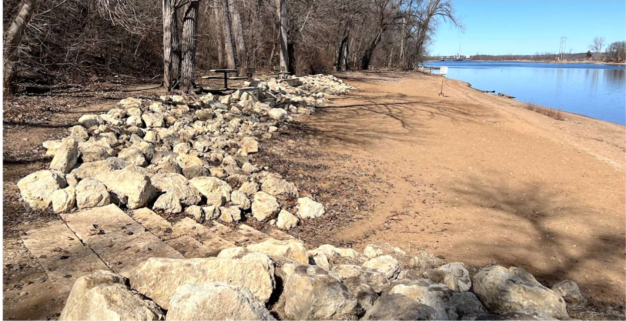
[Above] Lakeland Beach stabilization (October 2023).
