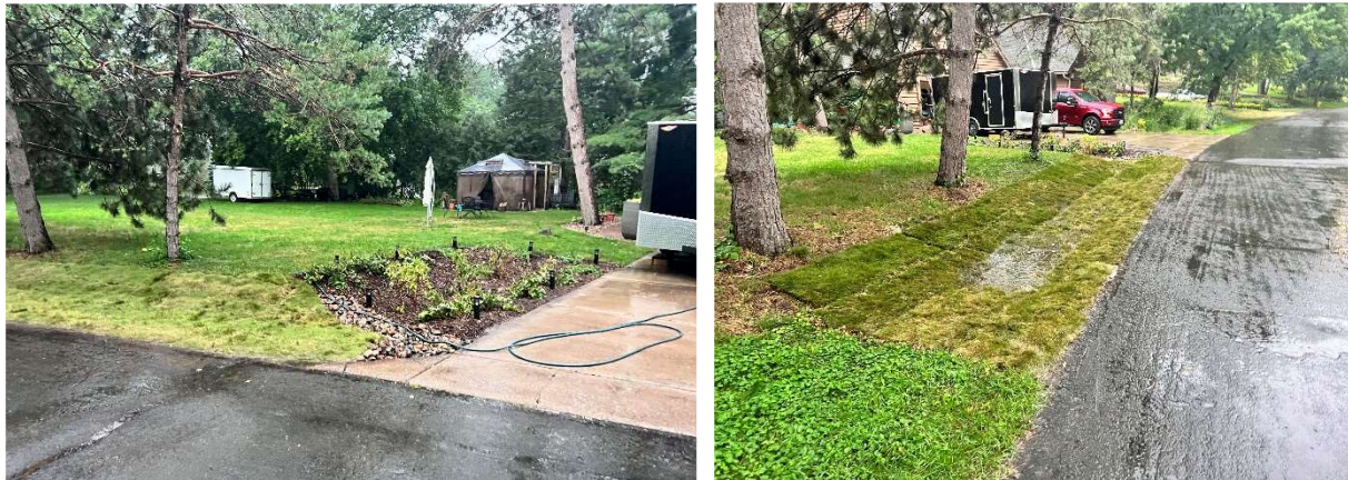
[Above] Riviera Avenue Treatment Train Bioretention.
